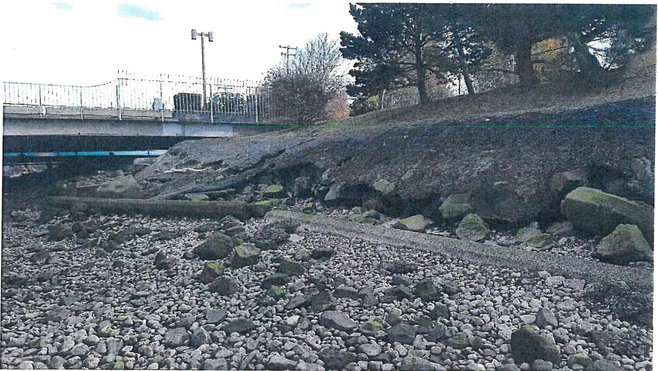
Photo 2 – Existing steep, erosional shoreline just landward of the SMA.
